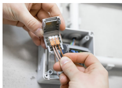
Place the wired connector in the Gelbox.
