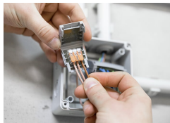
Place the wired connector in the Gelbox.
