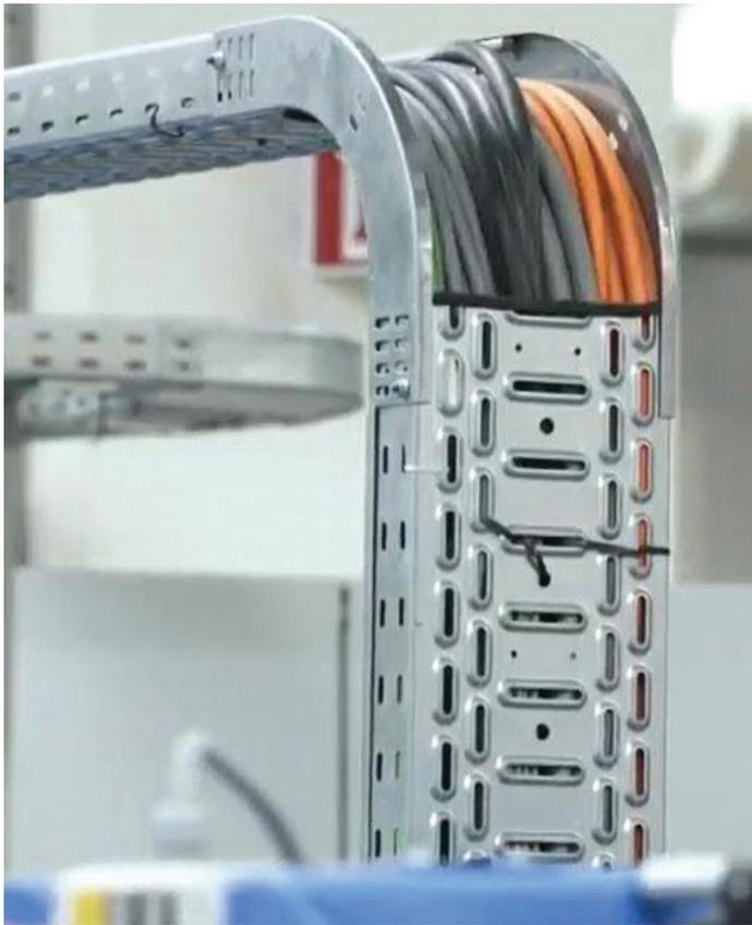
Along with being tray-rated, the ÖLFLEX SERVO FD 7TCE bend radius makes it ideal for tight corners.
